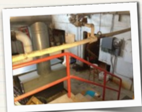
Boiler Room equipment dates to 1950s
